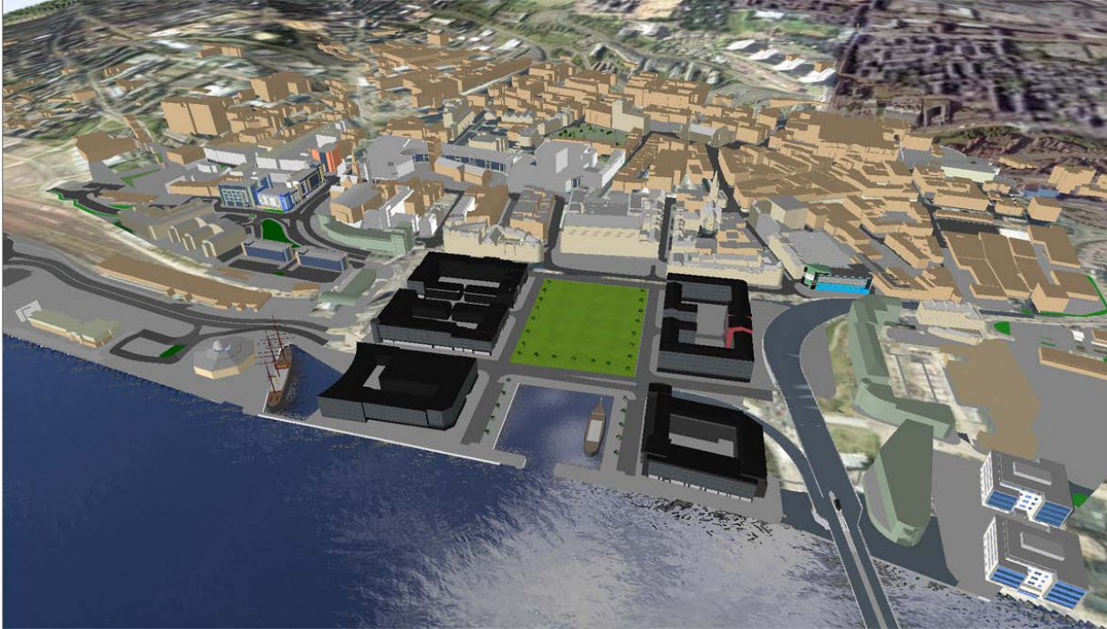
FIG. 3: 3D representation of proposed development within the city-wide context. The textured buildings in the centre of the image are consistent with the buildings created in designer view in Figure 1.
